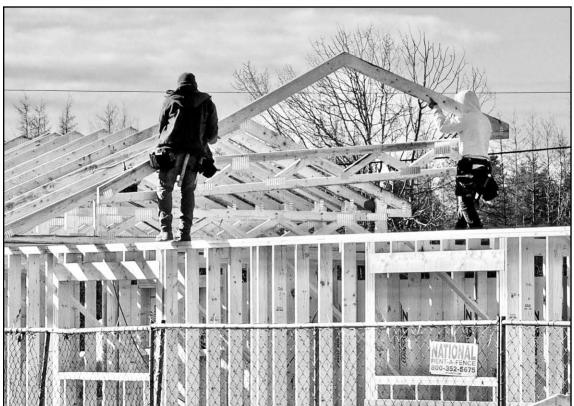
Thanksgiving Day was just another workday for this crew, installing roof trusses and outer wall panels on the recently framed Bluebird Motel on Outer Dublin Street in Machias. The new construction is going up on the exact footprint of the sections of the motel that went up in flames last year on Christmas Eve. (Photos by Paul Sylvain)
